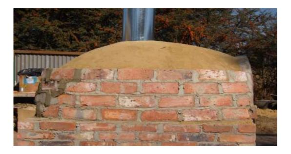
16. Continue by plastering the oven, and cork the brick arch's gaps that it can blend in with the plaster.
