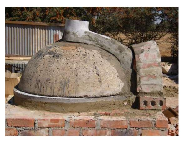
11. Place the smoke outlet behind the arch. It will naturally follow the contours of the dome. Small gaps between the dome and the smoke outlet and between the smoke outlet and the arch will appear. These gaps must be corked with normal dagga.
