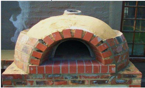
17. Once the plaster is dry the oven can be painted with normal PVA paint.
