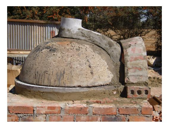
11. Place the smoke outlet behind the arch. It will naturally follow the contours of the dome. Small gaps between the dome and the smoke outlet and between the smoke outlet and the arch will appear. These gaps must be corked with normal dagga.
