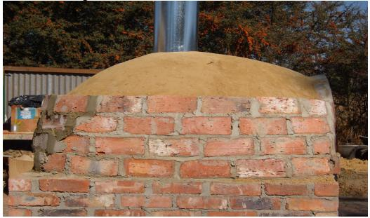
16. Continue by plastering the oven, and cork the brick arch's gaps that it can blend in with the plaster.
