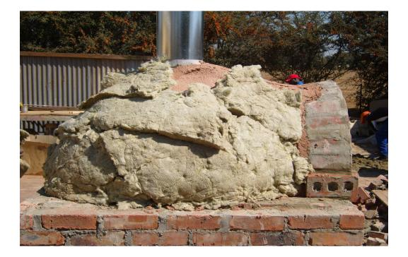
15. Start closing the oven by building and outer skin with clay bricks. Automatically a cavity will be formed witch gets filled with filling sand.
