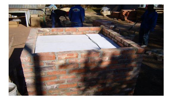
4. Construct this base with a solid concrete slab, 1m high from finished floor level.
