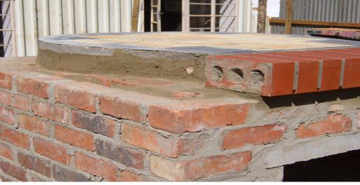
8. Install the brick sill in front of the oven, with the top of the sill level with that of the pizza ovens floor.
